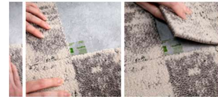
Tac-Tiles : Glue free carpet tile installation
