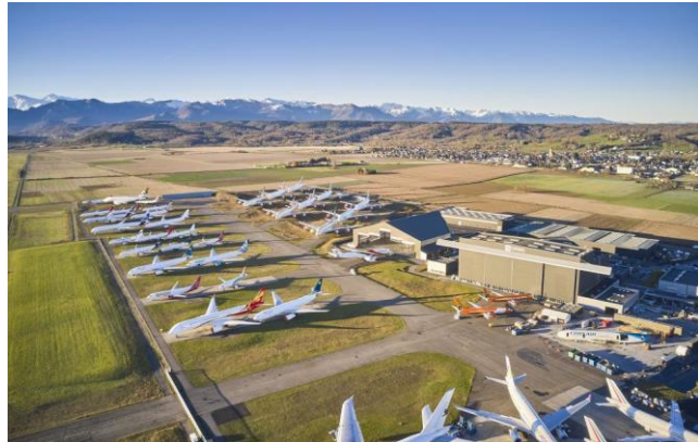
Picture of the TARMAC Aerosave site (Tarbes, France) where end-of-life aircraft are stored before being dismantled and
